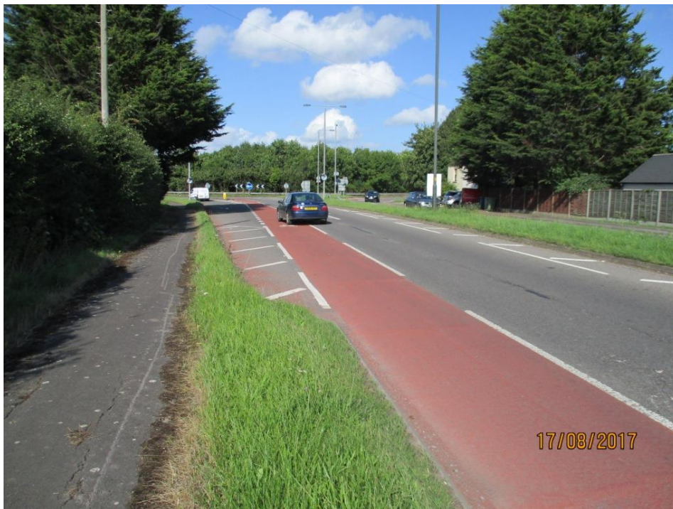
Photograph 9: Advisory cycle lane on A46, just west of the Shurdington Road junction
