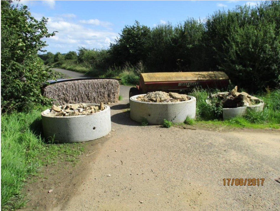
Photograph 2: Cycleway east of Birdlip
